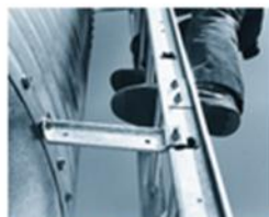
Side ladders allow plenty of space between rungs and bin wall for a secure footing.
