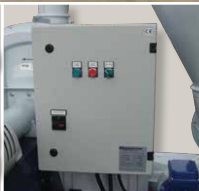
Control cabinet for automatic starting/stopping the motor.
