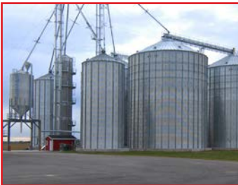
Grain Storage Bins
